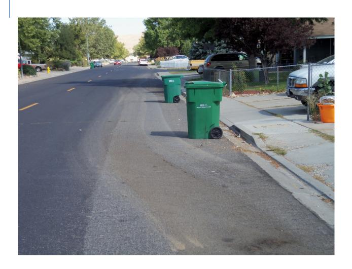
3 Gutter broom not in gutter, sweeping two feet away from gutter 10/04/2011.
