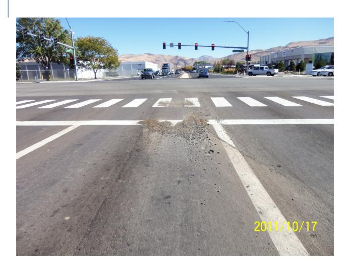
9 Sweeper picking up rear broom and leaving pile of material behind.
